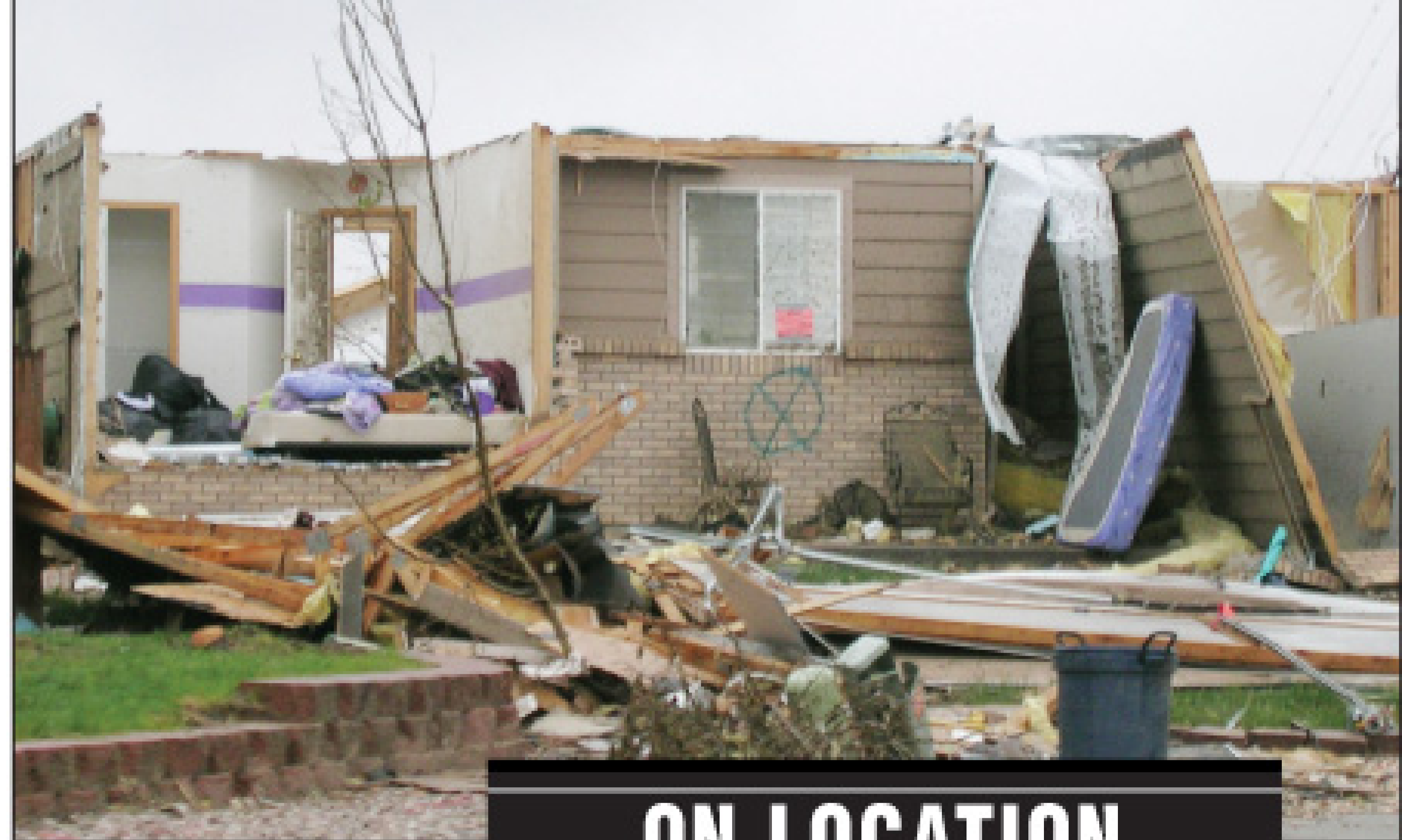
The need for portable restrooms was so great once reconstruction began that several companies were needed to supply them. At right: A home was destroyed by the tornado that touched down in May 2008. (Photos courtesy of Rebecca Valentine)
