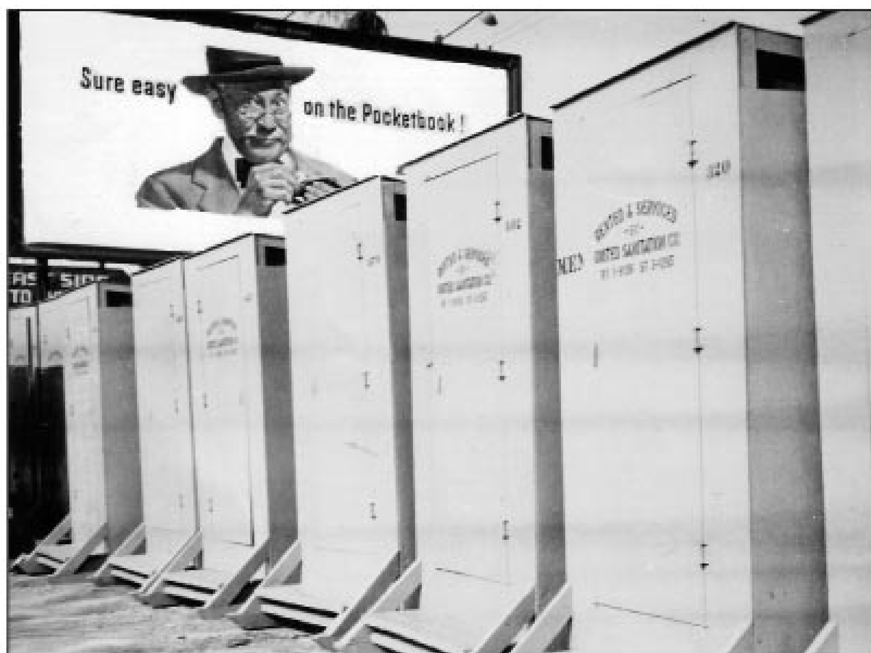
These were the first units Harvey Heather put out on jobsites, wooden models that weighed 500-600 pounds when filled to capacity.
