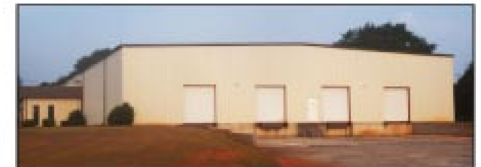
New 21,000-square-foot J & J Chemical plant.
