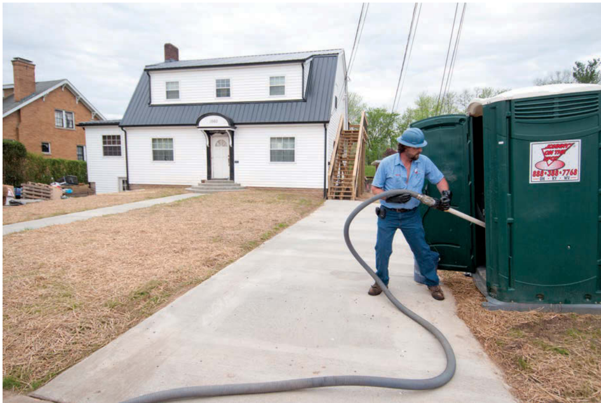
Technician Norm Anson pumps the holding tank of a construction unit in Ironton, Ohio.
