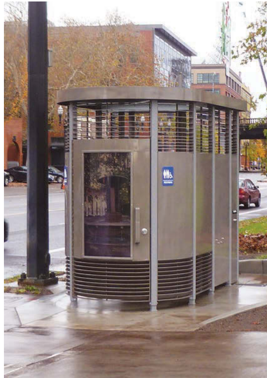
Right: The Portland Loo has a footprint of about 10 feet long and 6 feet wide with a rounded door on the front and an enclosed utility area in the back.
