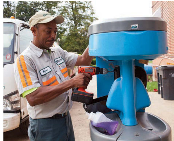
Below: Technician Myron Godbee secures a soap dispenser on a Satellite Industries hand-wash station.
