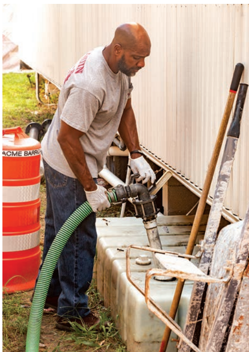
Above, Left: Fill Griffith pumps a 250-gallon holding tank (PolyPortables) at Florida State University's Doak Campbell Stadium in Tallahassee.
