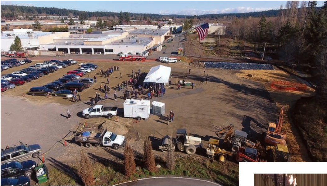
Left: A drone photo shows Randy-Kan Portable Restrooms' Satellite Suite restroom trailer and a Satellite / PolyPortables restroom serving the groundbreaking ceremony for a new VA hospital in Silverdale, Washington. (Photo courtesy of FPH Construction)
