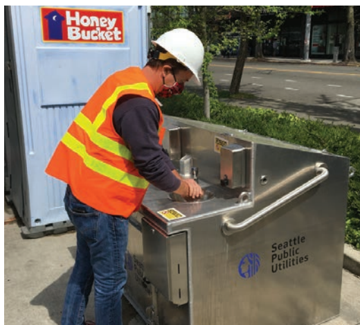
Left: A worker for Seattle Public Utilities is shown with a sink purchased for the city's hygiene stations. The unit is manufactured by University Mechanical Contractors and includes 100-gallon fresh and graywater tanks and 12-volt marine batteries to power push-button faucets and prevent freezing in winter.
