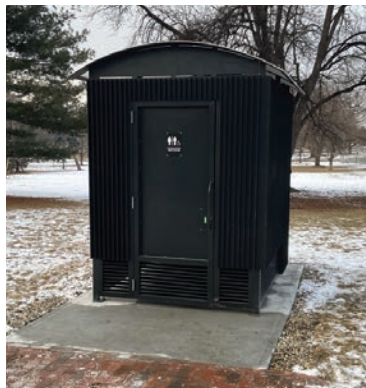
Above: One of the first units was bolted to a concrete slab in a park.
