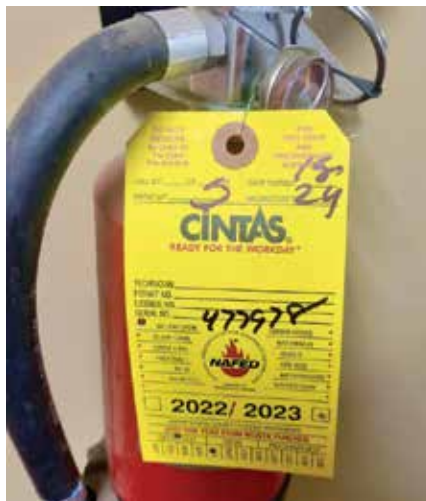
An inspection tag clearly shows the last date the fire extinguisher was tested.
