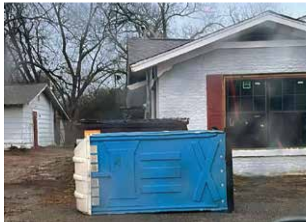
An unsecured restroom was tipped over on a construction site.
