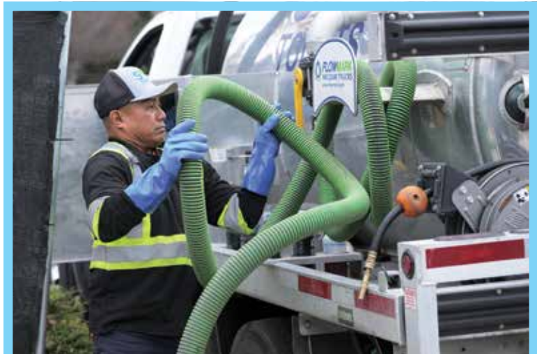
Above: Technician Rody Badua returns the suction hose after servicing a restroom at a home construction site. The truck is from FlowMark and carries a National Vacuum Equipment pump. Below: Badua pumps the holding tank of a NuConcepts trailer-mounted restroom unit stationed at an event in San Jose, California. The International service truck carries a National Vacuum Equipment pump and was built out by FlowMark.
