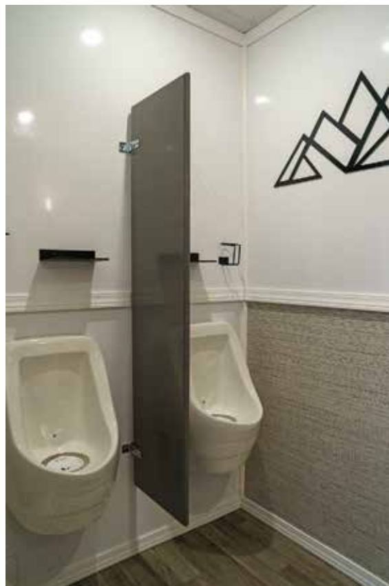
Urinals with a divider on the men’s side provide some privacy while allowing lines to move more quickly.
